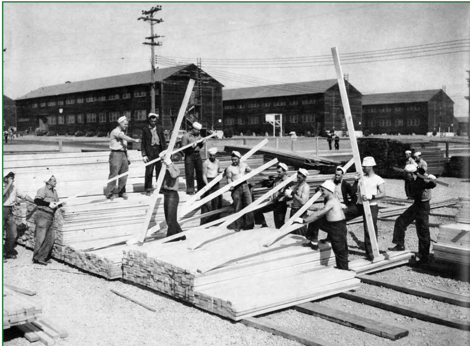
Seabees expanding the massive Camp Parks complex. NHC
