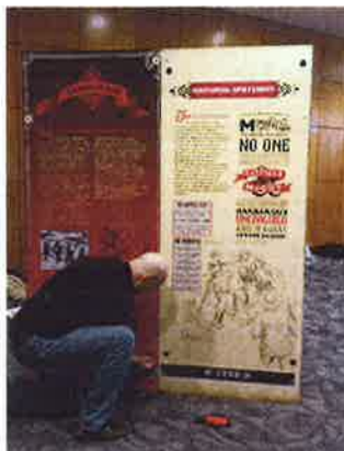
Add final panel. Bolts are tightened from both inside and out.
