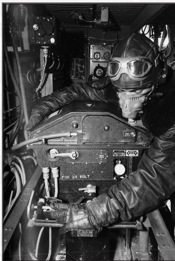
A VD-1 photographer prepares an aerial mapping camera rig in the bomb bay of one of the squadron’s PB4Y-1 Liberators. US Navy photo
