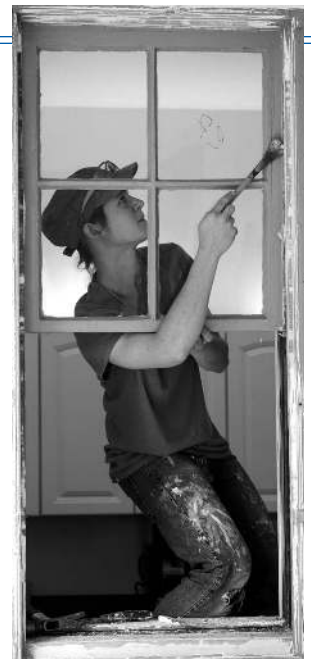
Nikkita Carin of Allegheny Restoration at work.
