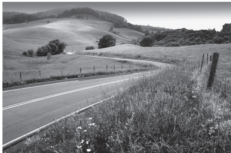
Route 50, outside of Grafton, Taylor County, WV
